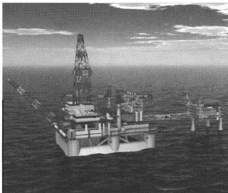
Fig. 1 Complex of offshore facilities for Korchagin Field
